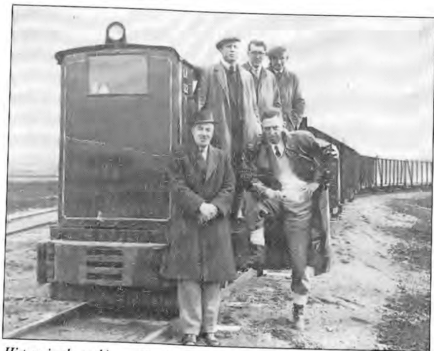
History in the making ... The first delivery of milled peat to Ferbane Power Station in 1957 was an historic occasion. On hand to witness the event were D.C. Lawlor, General Manager and C.S. (Todd) Andrews, Managing Director. Behind are key Boora personnel Hubert Collins, Bog Foreman; Tom Quinn, Civil Engineer and Christy Doolin, Transport Foreman.
