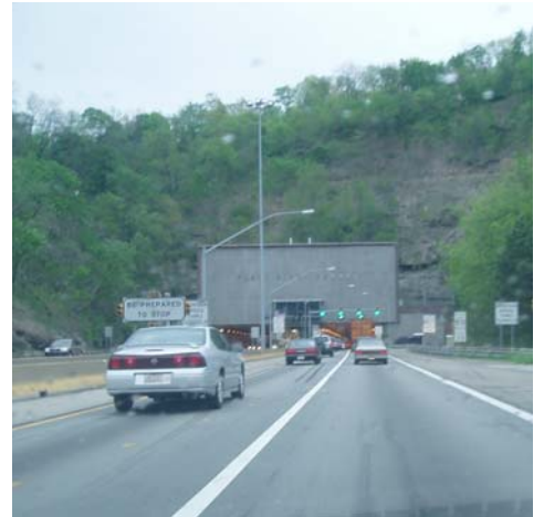
Fort Pitt Tunnel South Entrance
