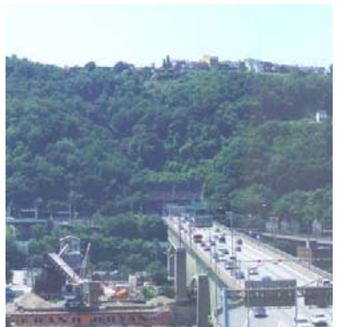
Liberty Bridge and Tunnel Entrance
